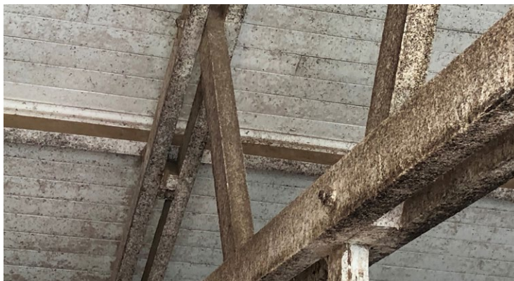
Image 1: Heavy fly spotting (droppings) on roof trusses
