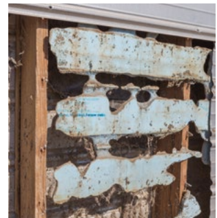
Rodents damage your facility in many ways from gnawing on electrical wires and destroying insulation.
